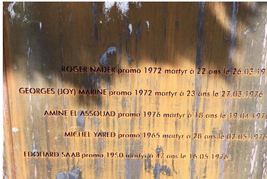
Memorial Wall at Collège Notre-Dame de Jamhour Architect: AAA Atelier des Architectes Associés Contractor: Isotech S.A.L Description: Laser cut COR-TEN A weathering steel
